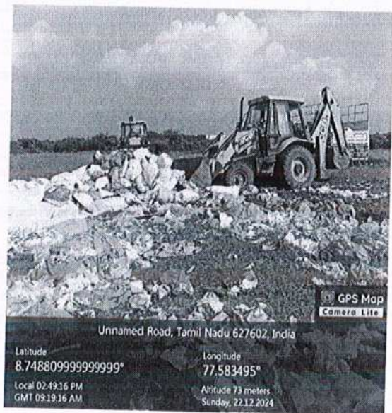
Removing waste from Heap No.3
