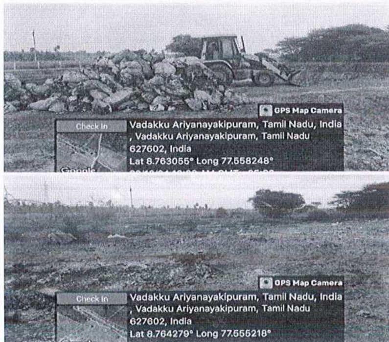
Site condition - before and after
