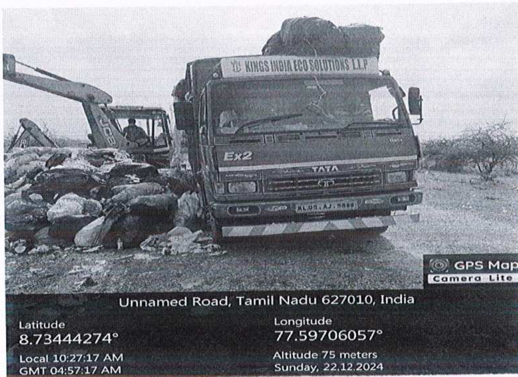
Loading into trucks
